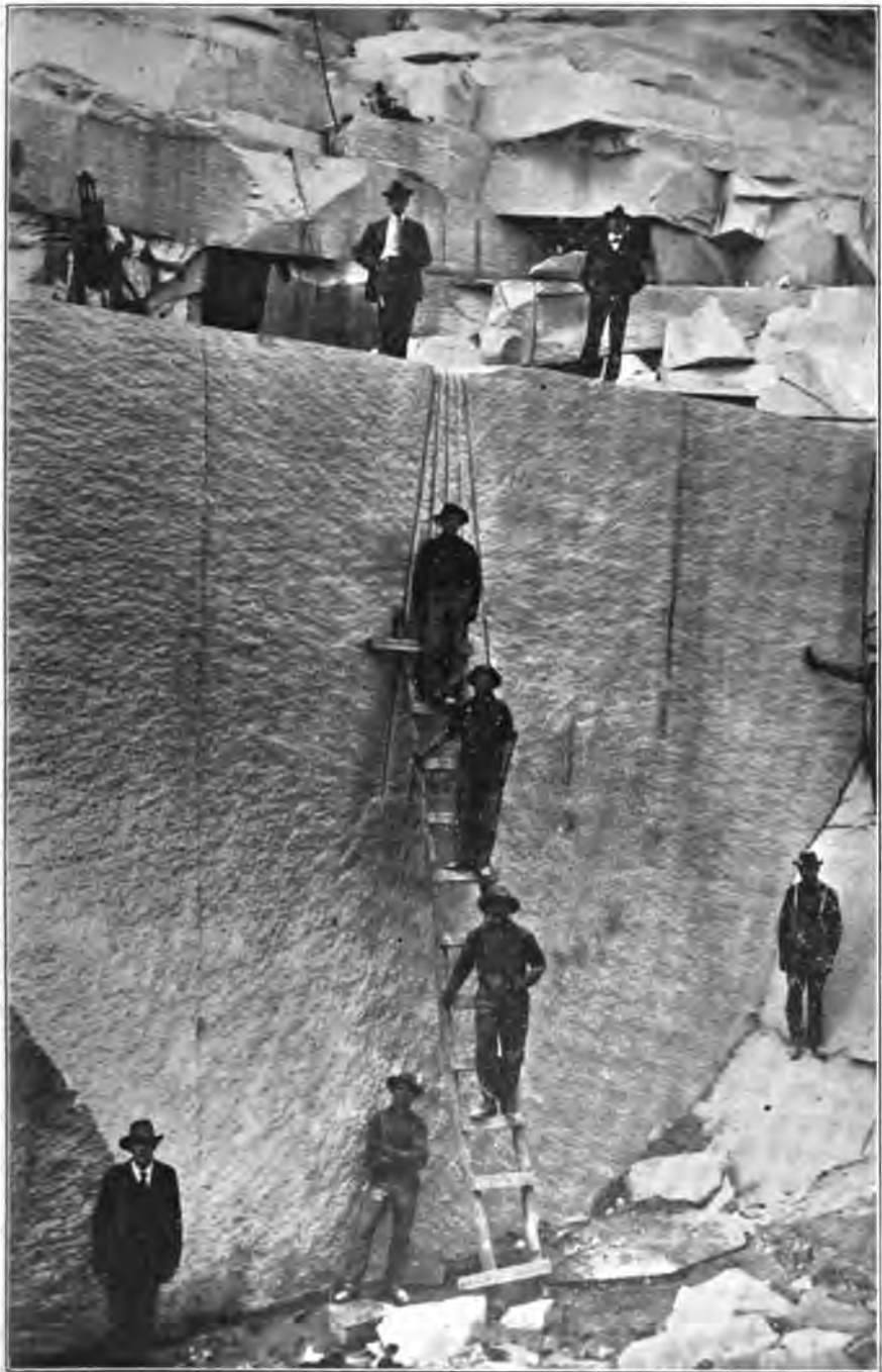
Section of a sheet 28 feet thick in the quarry of the Wetmore & Morse Granite Company at Barre, Vt.
